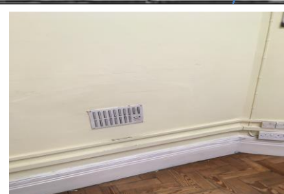
Replace existing vent with larger version.
