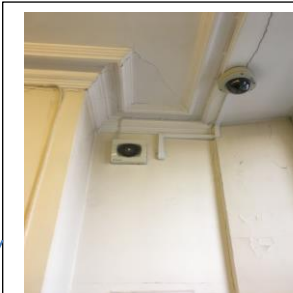
Existing Extract only fan to be replaced with new supply mode fan.
