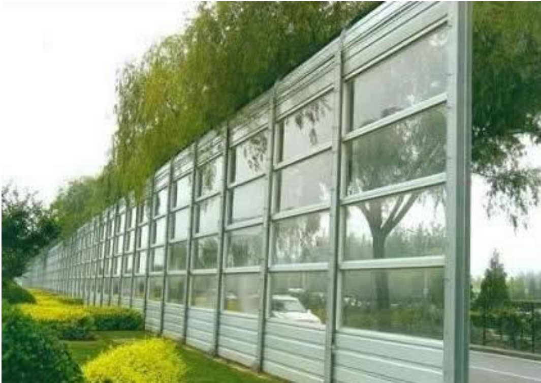
Example of the original clear acrylic acoustic screen system. (Currently unavailable)
