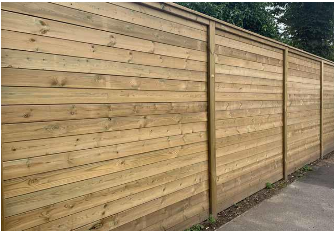
Example of an acoustic timber fencing system (substantially lower than proposed).
