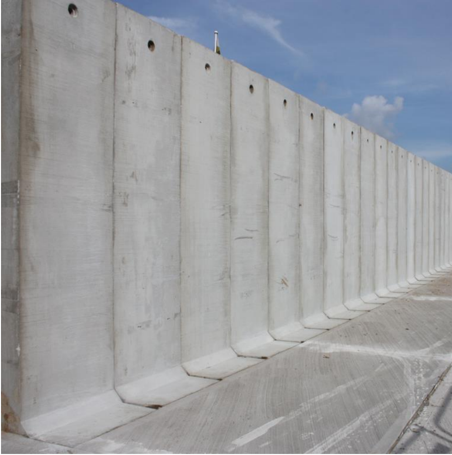
Example of a pre-cast concrete screen walling system.
